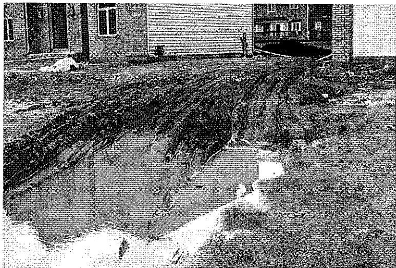
FIGURE 2. Heavy equipment on construction sites often destroys soil structure, resulting in poor water drainage.
